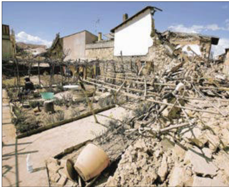
We know something can happen to threaten our business at some time. It could be a natural disaster - earthquake, hurricane, fire or flood. REUTERS
